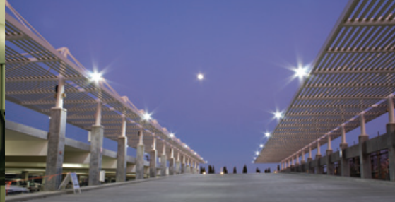
South Entry Parking Structure, 2009
