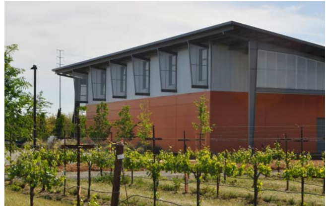
The Jess S. Jackson Sustainable Winery Building
