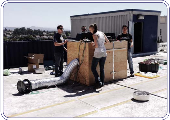
WCEC engineers utilizing a testing apparatus to measure the flow rates through the exhaust shaft of a multi-family building.
