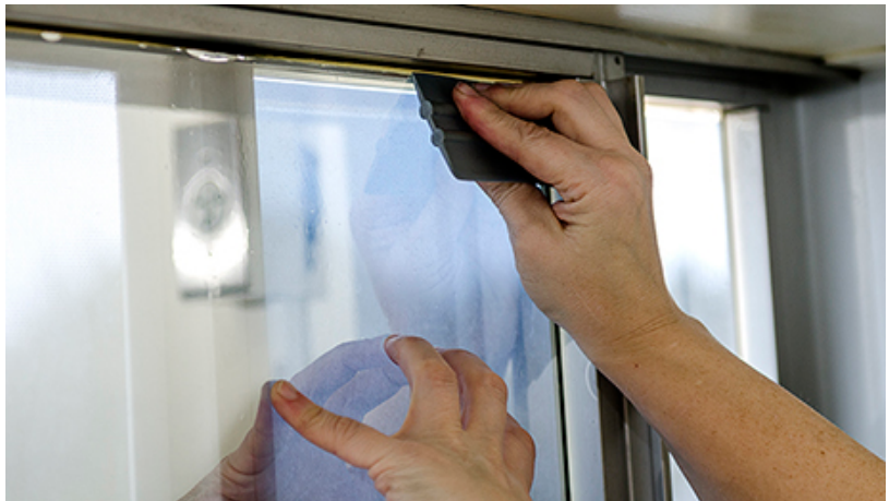
Figure 1: Window film being installed (source: http://ipf.msu.edu/green/practices/reflective-window-film.html )
