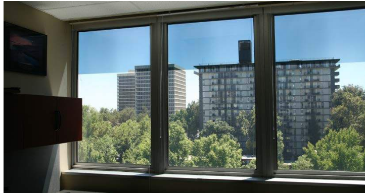
Figure 1: Electrochromic windows with sub-pane zoning. The upper part of the windows is tinted in order to provide glare control; the lower part of the windows is clear in order to provide daylight (source: LBNL).
