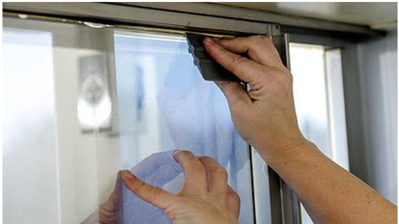
Figure 1: Window film being installed (source: http://ipf.msu.edu/green/practices/reflective-window-film.html )
