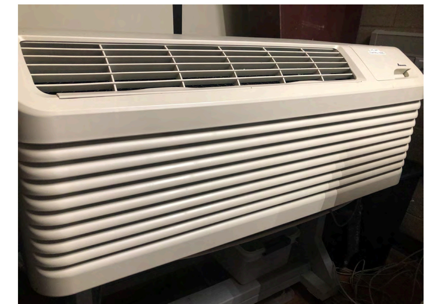
Figure 7. HVAC unit used in laboratory testing to confirm communication with integrated system components
