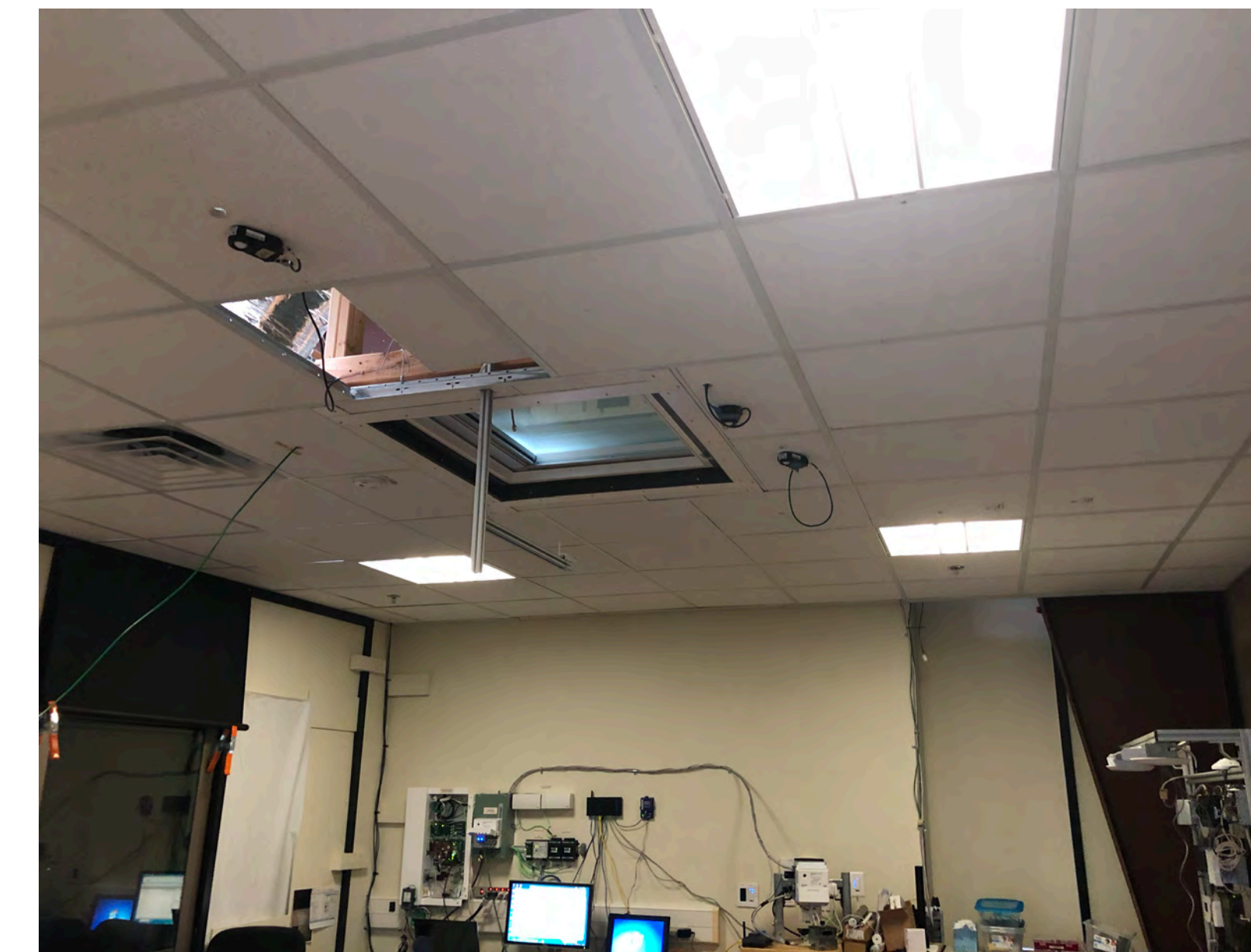
Figure 4. Electric lighting system in CLTC laboratory
