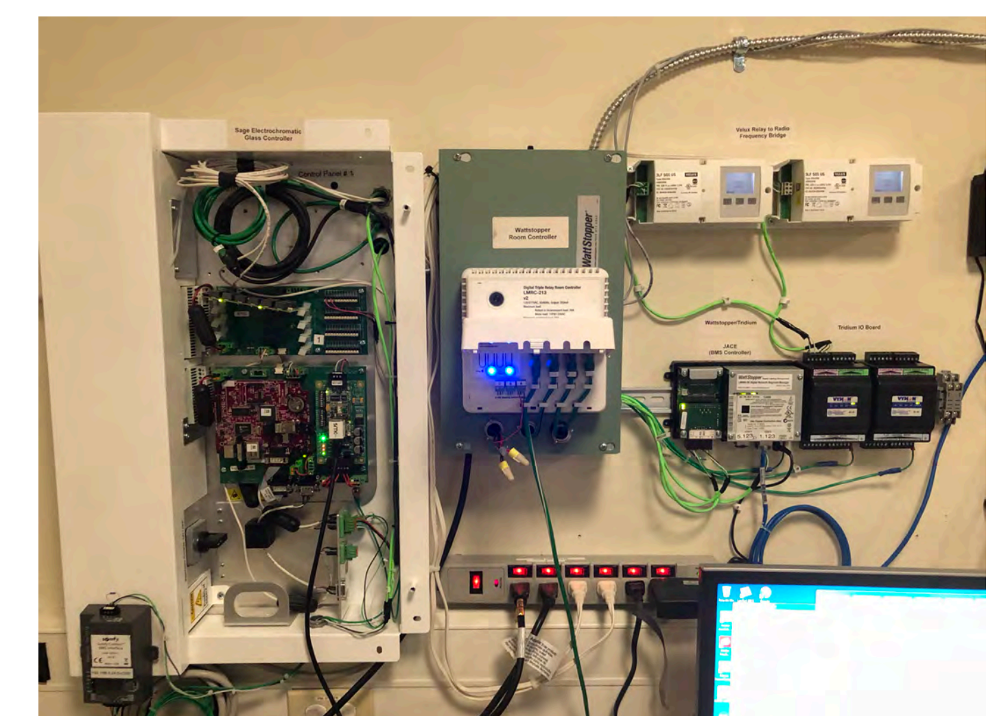
Figure 8. Automated Controls: Central controller and system controllers for IBCRP
