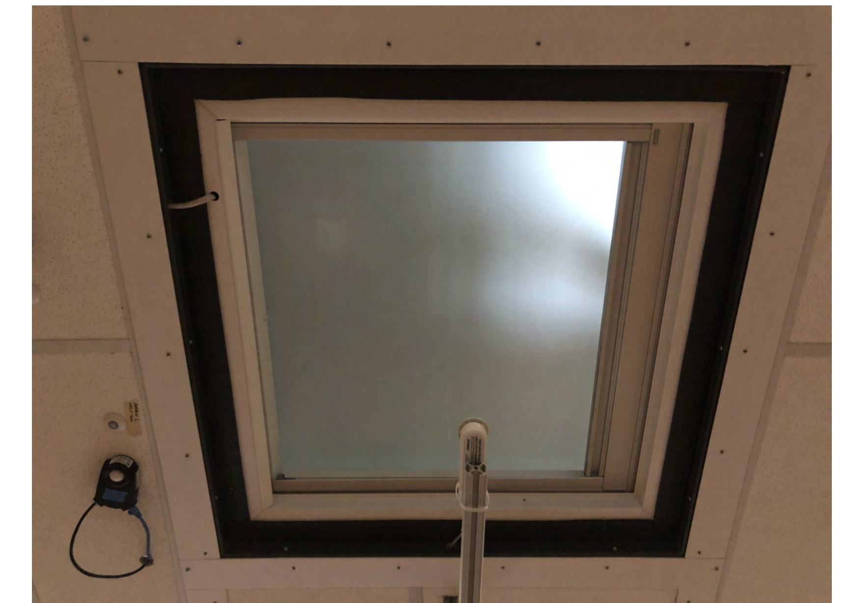
Figure 5. Venting skylight with solar shade and photo sensor looking outdoors.
