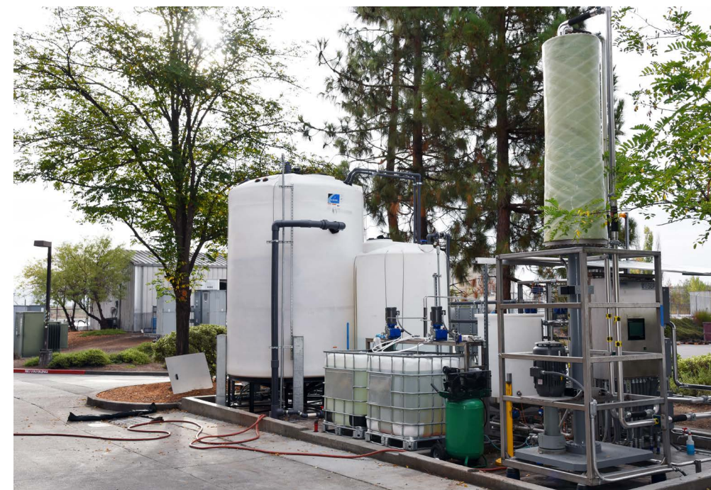
VSEP water recycling technology demonstration at the winery
