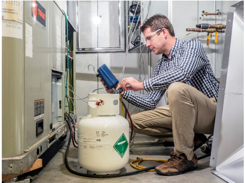
Figure 1: Technician charging a system with refrigerant
