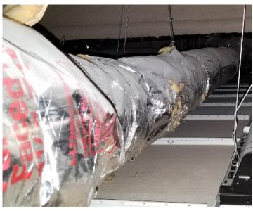
Measured Supply Leakage downstream of two VAV boxes with ASHRAE Std 215 = 12-30%
