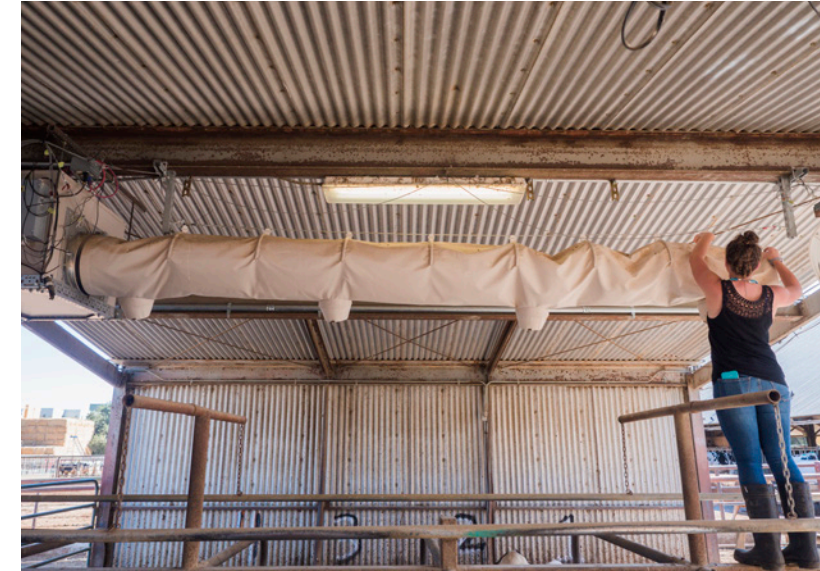
Installation of the convection cooling duct system and direct evaporative cooler
