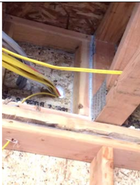
Seal formed at rim joist
