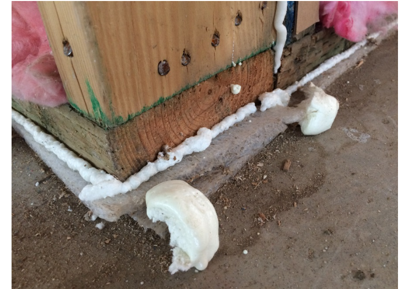
Can foam and gasket at sill plate
