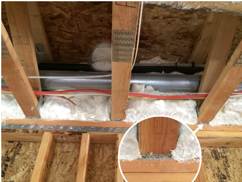
Seals formed under trusses
