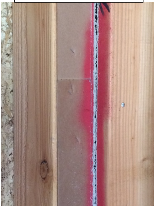
Seal between studs
