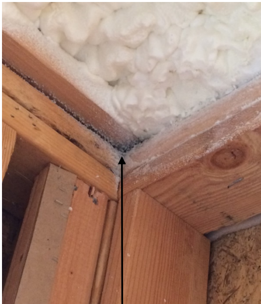
Seal formed at corner of wall assembly
