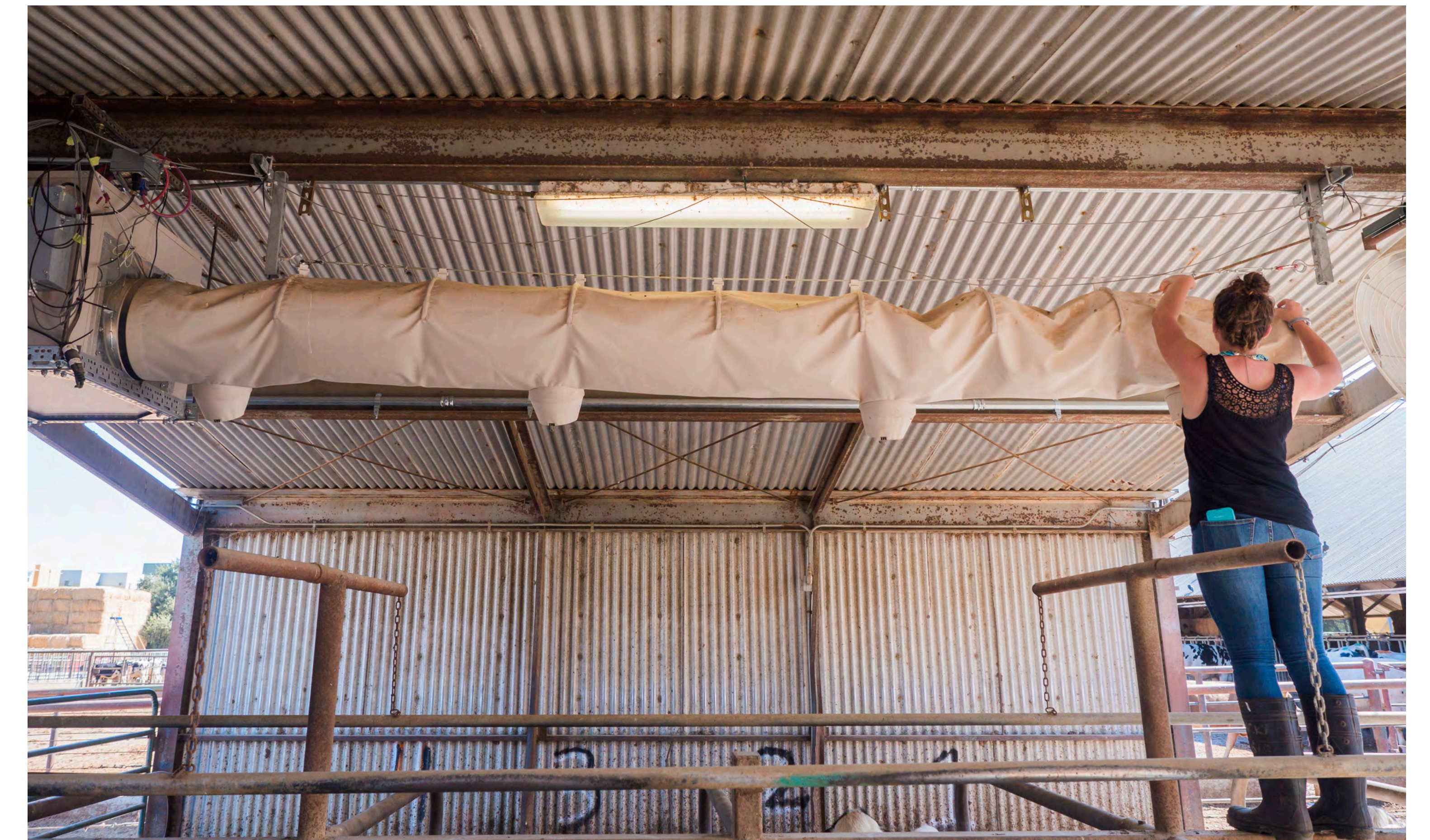
Installation of the convection cooling duct system and direct evaporative cooler
